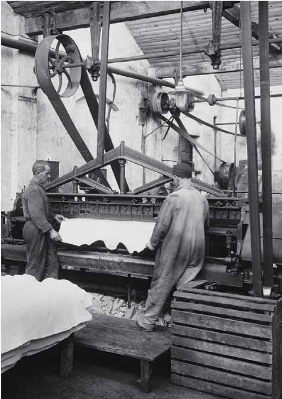
Splitting or levelling the hides done at Conceria Chiorino with the help of an American-made Turner machine (circa 1930).
